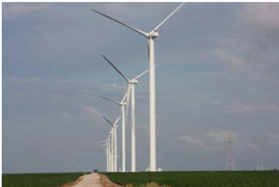
SJC becomes the largest private landowner with the most windmills east of the Mississippi River
